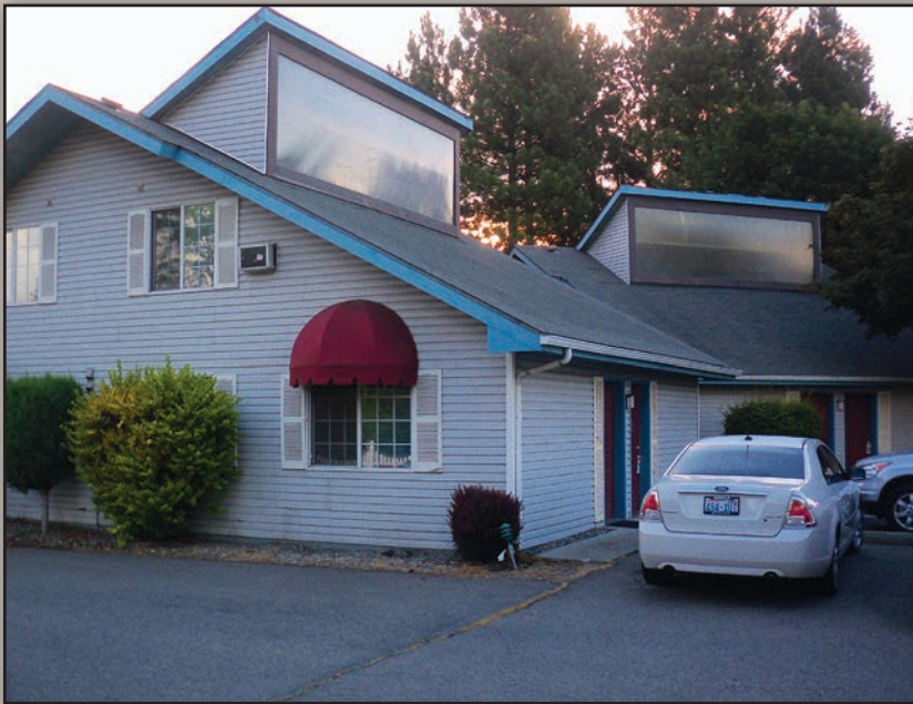
Top: Solar World Estates West was constructed between 1987-1990 with 94 units in 24 four-plex buildings
