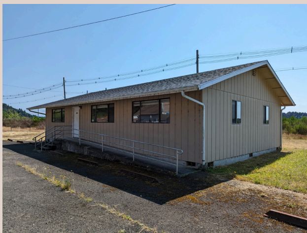
LP&N Office Building
