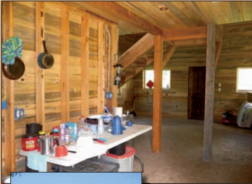
Kitchen area is ready to be finished
