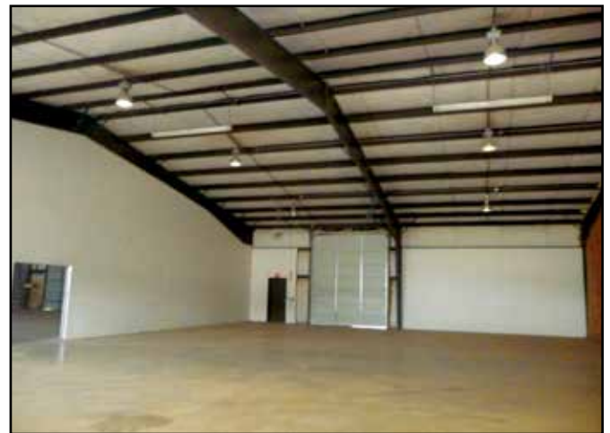
Interior bay of Building B
