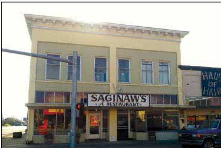
Auction Property #19 – Building in downtown Elma
