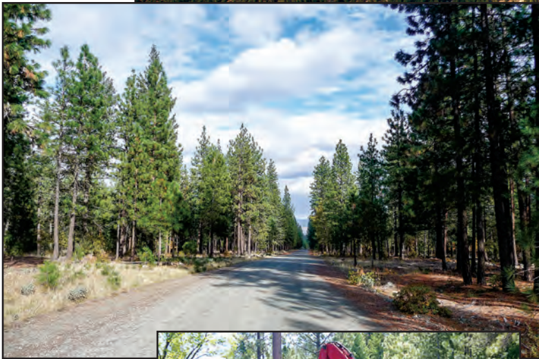
North entry road to Scott Valley North Block
