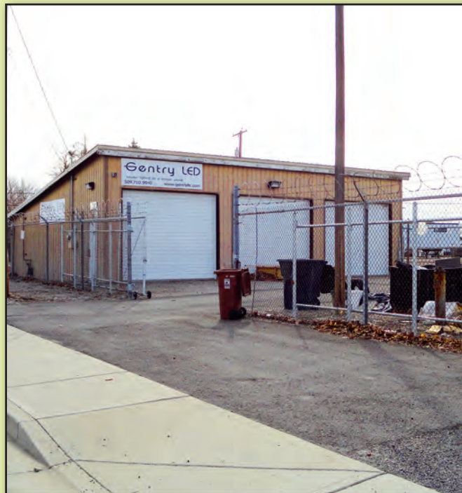
Left: Building One, 3,612± sq. ft. with office/ warehouse
