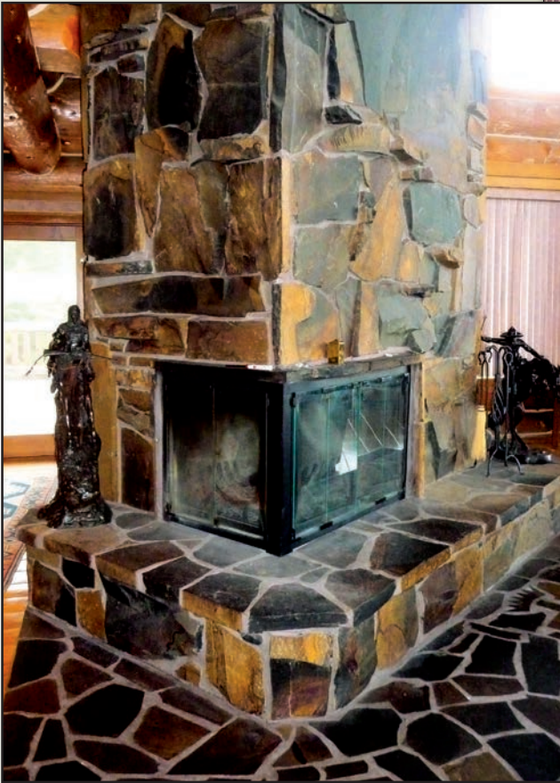
Two level stone masonry fireplace
