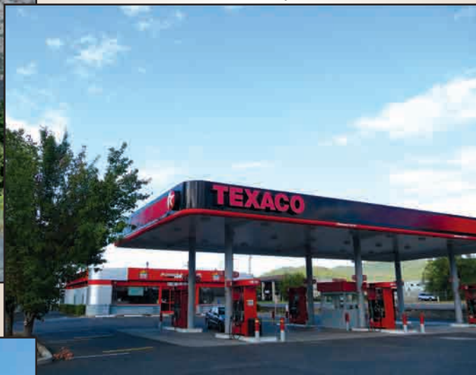
Gas station/C-Store/Car wash by retail center near I-5
