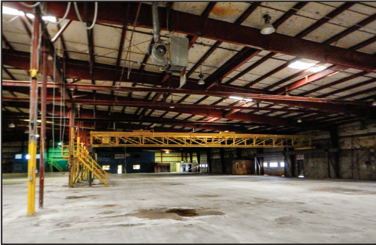
2 two-ton cranes are part of sale
